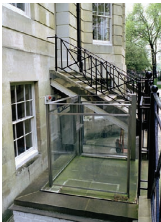
King's Bench Walk, Inner Temple, London. A short-rise platform lift is positioned behind railings where it descends to basement level and connects to the primary circulation routes.
