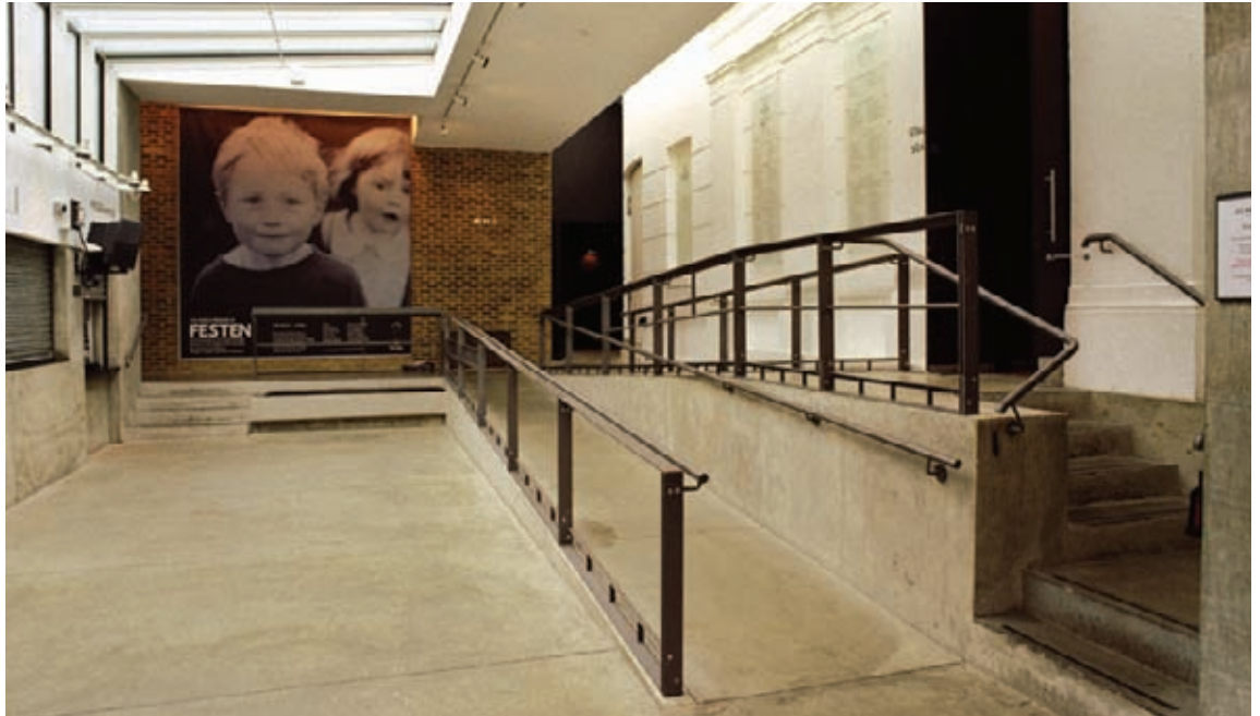
Access improvements at the Almeida Theatre, London, were part of a larger project. The foyer ramp gives access to the stalls seating area.
