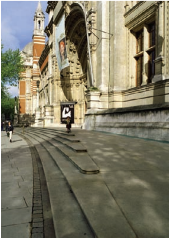
At the Victoria and Albert Museum in London long symmetrical shallow ramps have been combined with steps that complement the scale of the Cromwell Road frontage. There is one central handrail to the steps.
